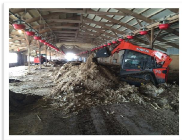
Constructing the core (photo by Bob Peer)
