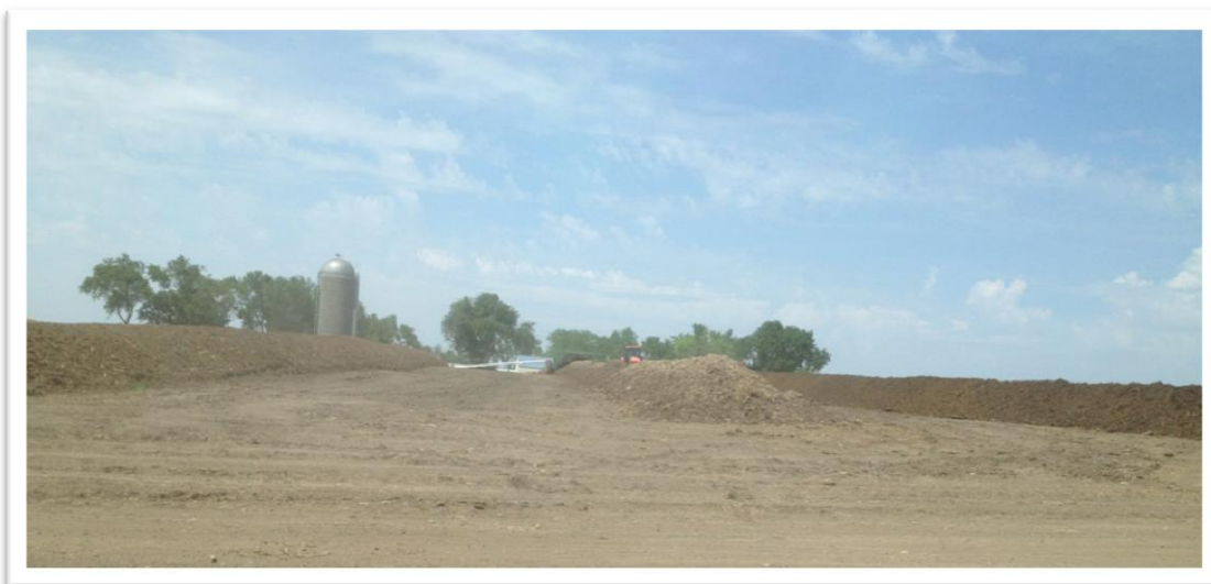
HPAI compost site (photo by Mark King)
